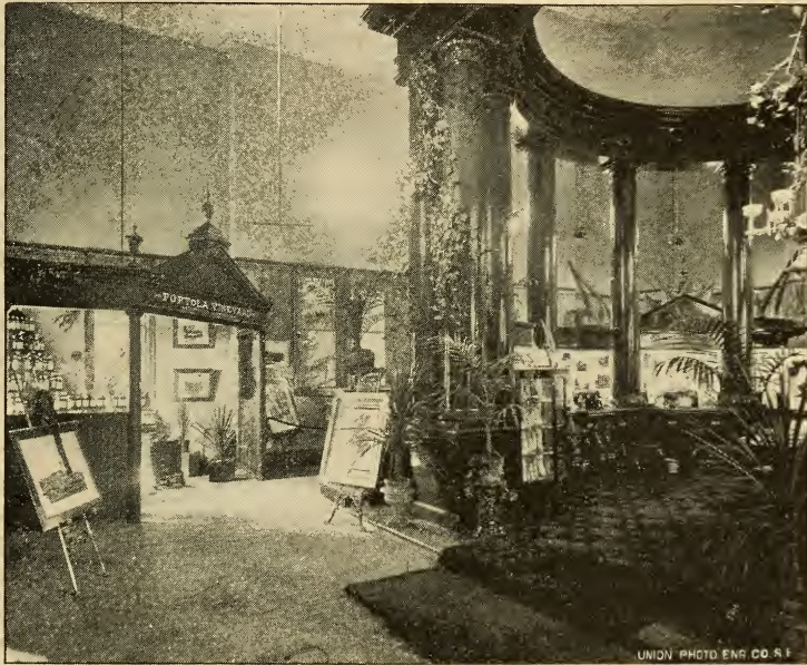
SAN MATEO COUNTY BUILDING—INTERIOR
